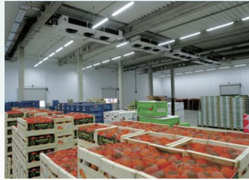
Fig. 6.1: Cold Storage Facility
